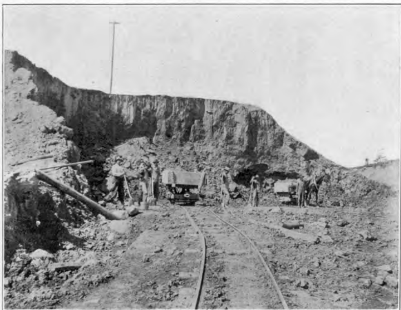
Fig. 2. Bank of Manitowoc Clay Mfg. Co., Manitowoc. The clay is worked by falling and the run of the bank is used. It is loaded on cars which are hauled to the yard.
