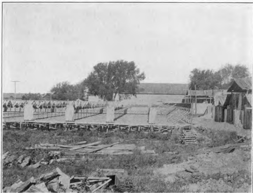
Fig. 1. Drying racks at Whittet's brick yard, Edgerton. The bricks are dried on the racks, which can be covered by canvas screens to prevent rapid drying and cracking.
