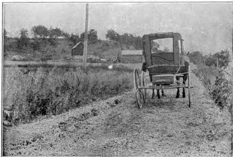
Fig. 2. Sand road freshly covered with straw
