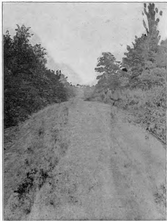
Fig. 2. Same road showing the effect of use of the "split-log" drag.
