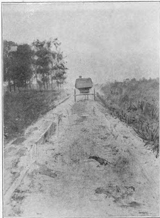
Fig. 1. Clay road in Calumet county with shallow ruts filled with water just after a shower.
