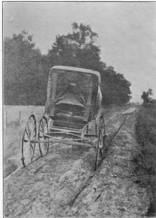
Fig. 2. More heavily traveled clay road one-half mile from road at left showing effects of allowing water to stand in ruts.
