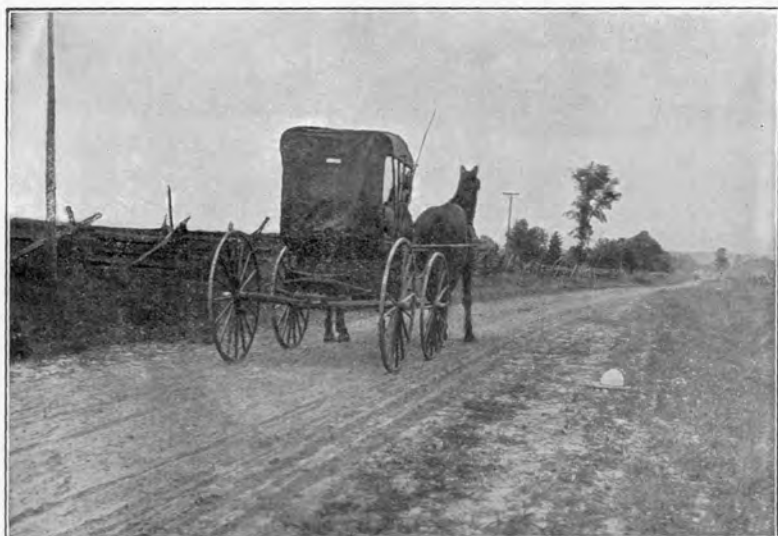
Fig. 1. A flat-topped clay road in Clark county. The ruts appearing in the picture are wheel tracks in a thick layer of dust.
