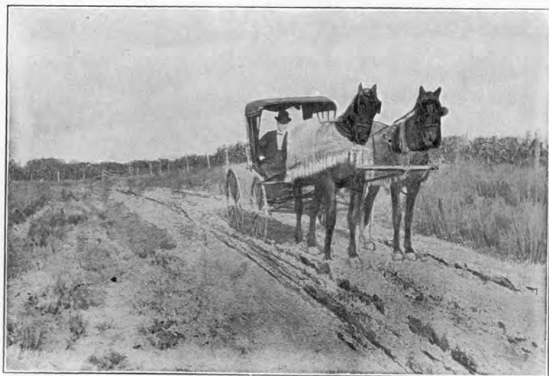
Fig. 2. Flat-topped clay road in Clark county showing how such a road ruts when wet.
