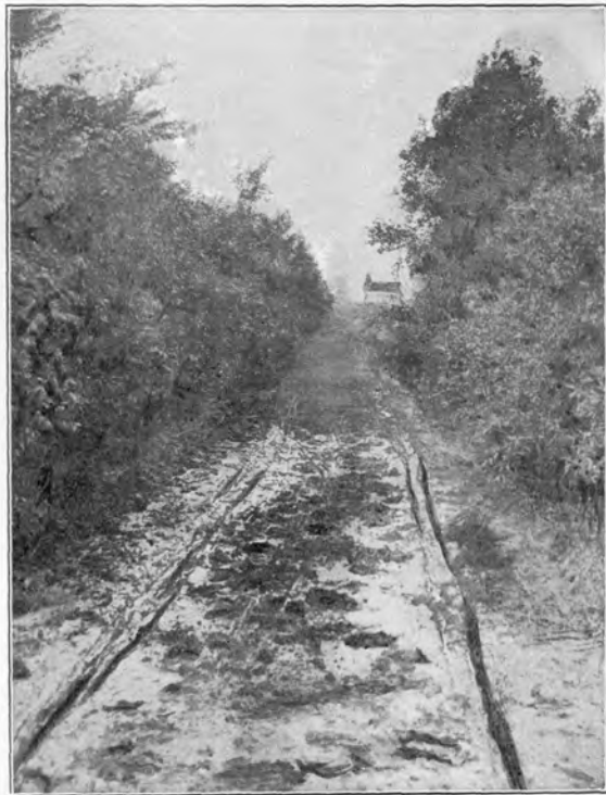
Fig. 1. Road in Waupaca county. Low place which has not yet been graded and dragged with the "split-log."
