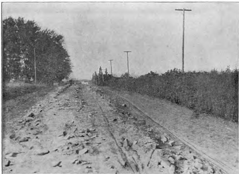
Fig. 1. Sandy road in Trempealeau county covered with shale, in which the sandstone was left in large pieces.
