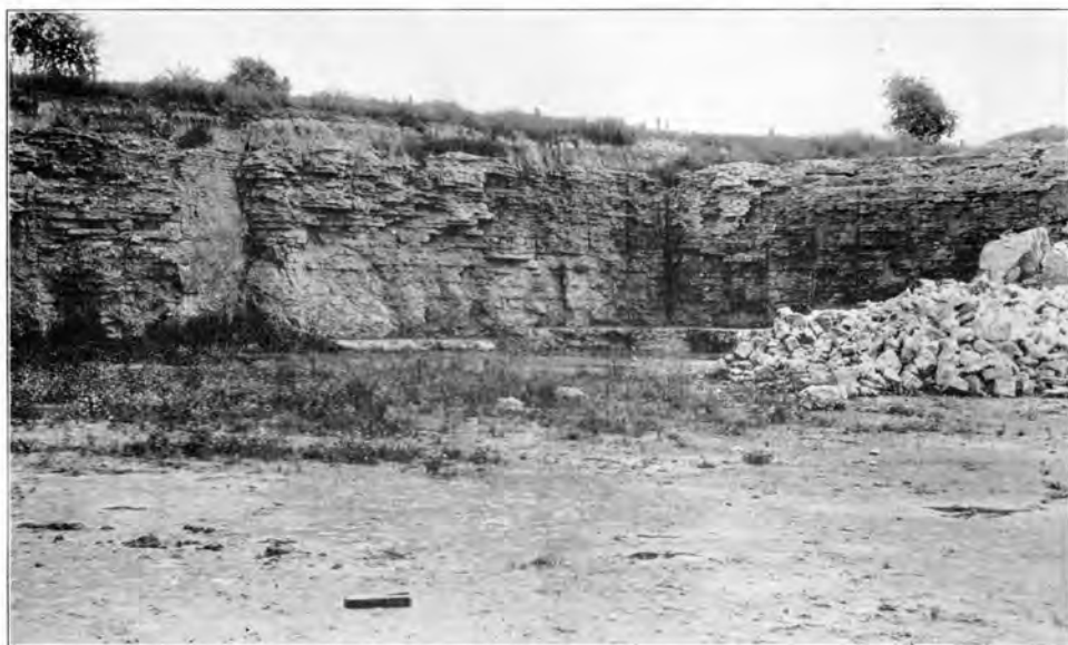
Whitewater city quarry. Flat-lying layers of Trenton limestone, a uniform but rather mediocre road material. The quarry faces are parallel to joint planes which cut the rocks in two directions at right angles to each other.
