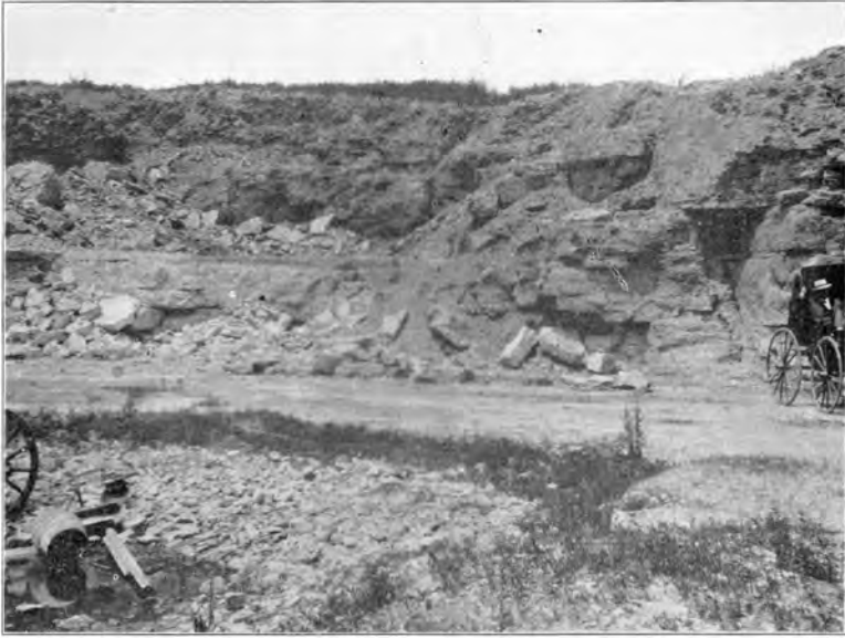
The McGavock quarry near Janesville. The lower beds of this quarry are compact and of fair quality for road construction. The upper beds are broken into a rubble by frost action and grade into the soil which overlies them.
