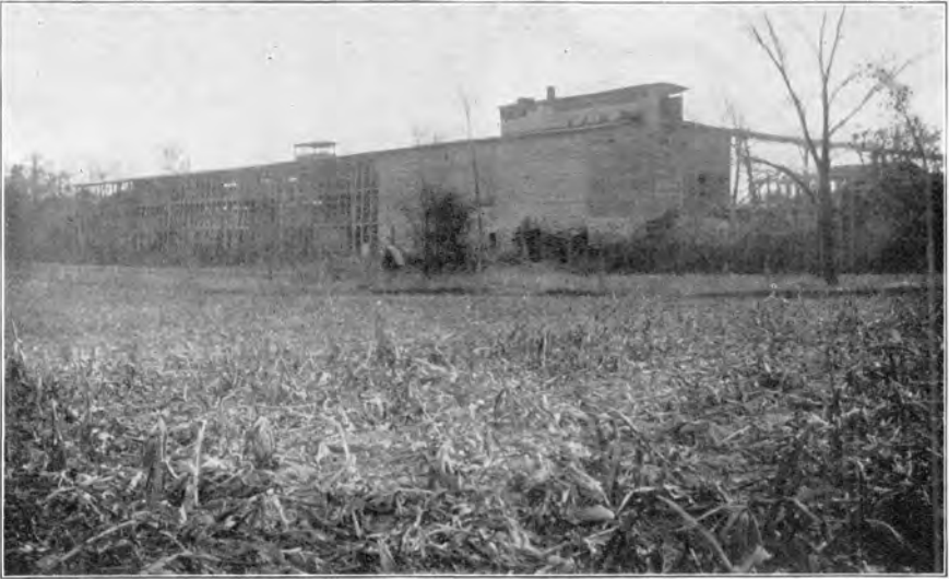
THE FACTORY OF THE LAMARTINE PEAT, LIGHT AND POWER COMPANY (EXTERIOR VIEW) FOND DU LAC, WISCONSIN
