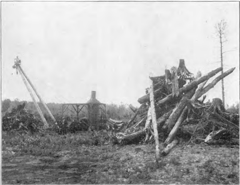
FIG. 2 THE STEAM PULLER WITH THE ATTACHMENT FOR PILING STUMPS IN HUGE HEAPS.
