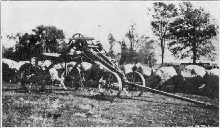
AN IMPLEMENT FOR LIFTING AND REMOVING LARGE BOULDERS.
