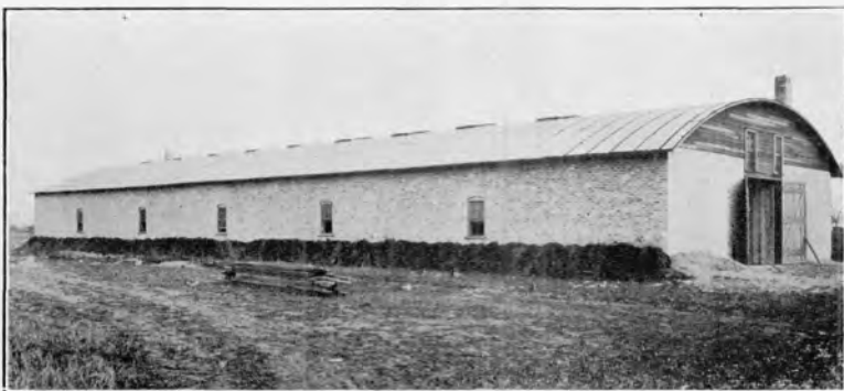
A well constructed storehouse on a truck farm in southeastern Wisconsin. Such buildings are used for storing such crops as cabbage, onions, etc.
