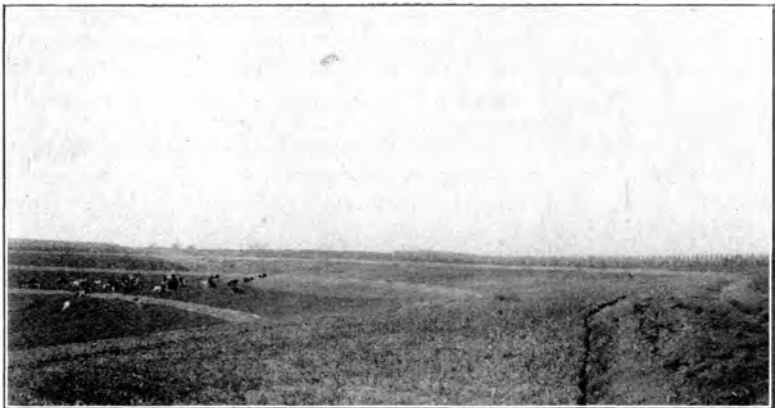
Fig. 7. Terraces constructed on moderately sloping land to prevent erosion.
