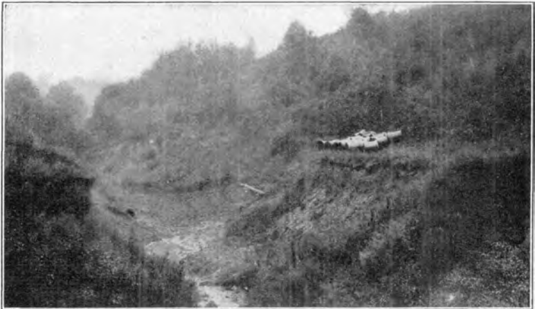
Fig. 5. Upper side of dam in gully just made to cause filling of gully. The tile through the dam will be extended upward as the gully fills.
