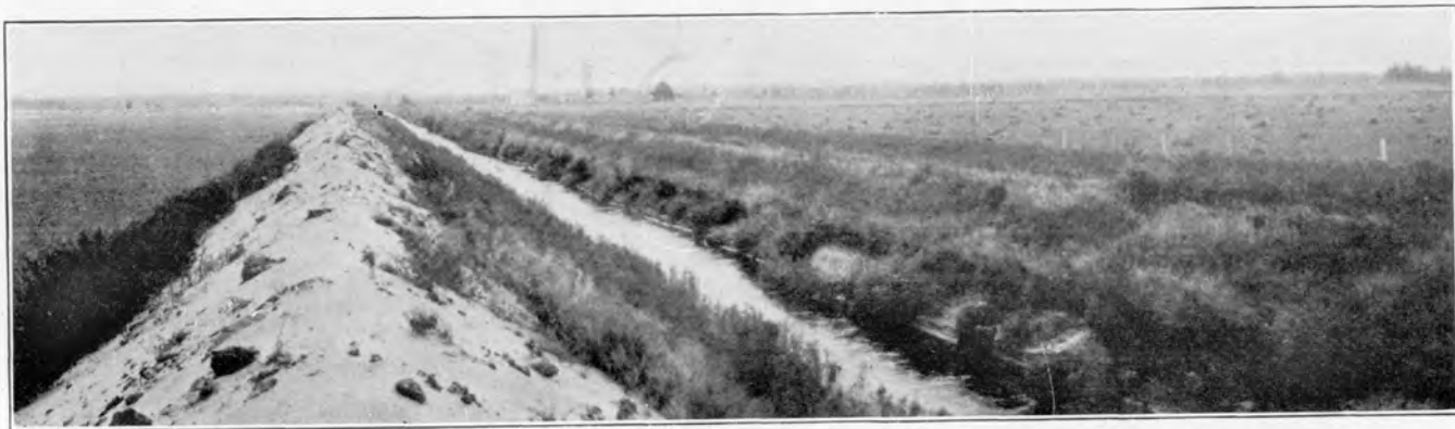
Plate XX-B. Drainage ditch through peat marsh in central Wisconsin showing sand underlying peat.
