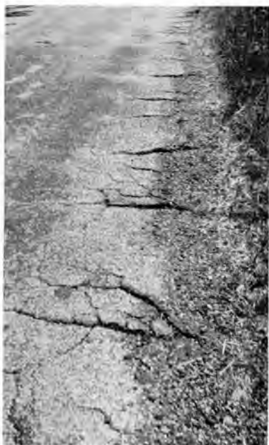
Figure 8. Cracks in pavement indicate failure of the poorly drained underlying silty soil to provide stable support in seasons of high water table and frost action.
