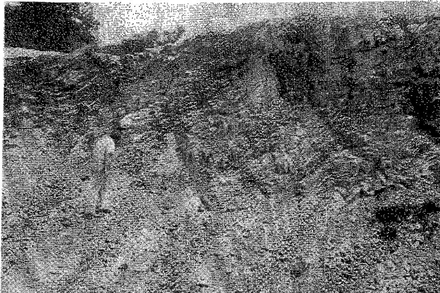
Figure 26. Excavation face at Hamilton Mound showing steeply dipping beds in quartzite cut by nearly horizontal fracture cleavage.
