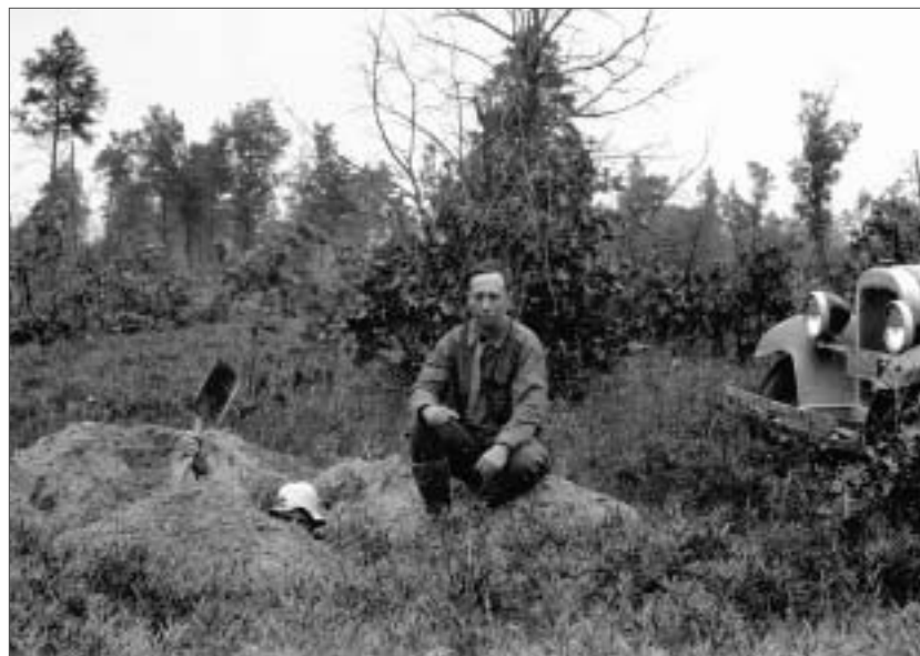
Figure 6. F.T. Thwaites at test pit searching for red drift as part of road materials survey, 8 miles northeast of Shawano; assistant's hat, hand, and shovel are sticking out of pit. WGNHS photograph 4284, by F.T. Thwaites, July 25, 1928.
