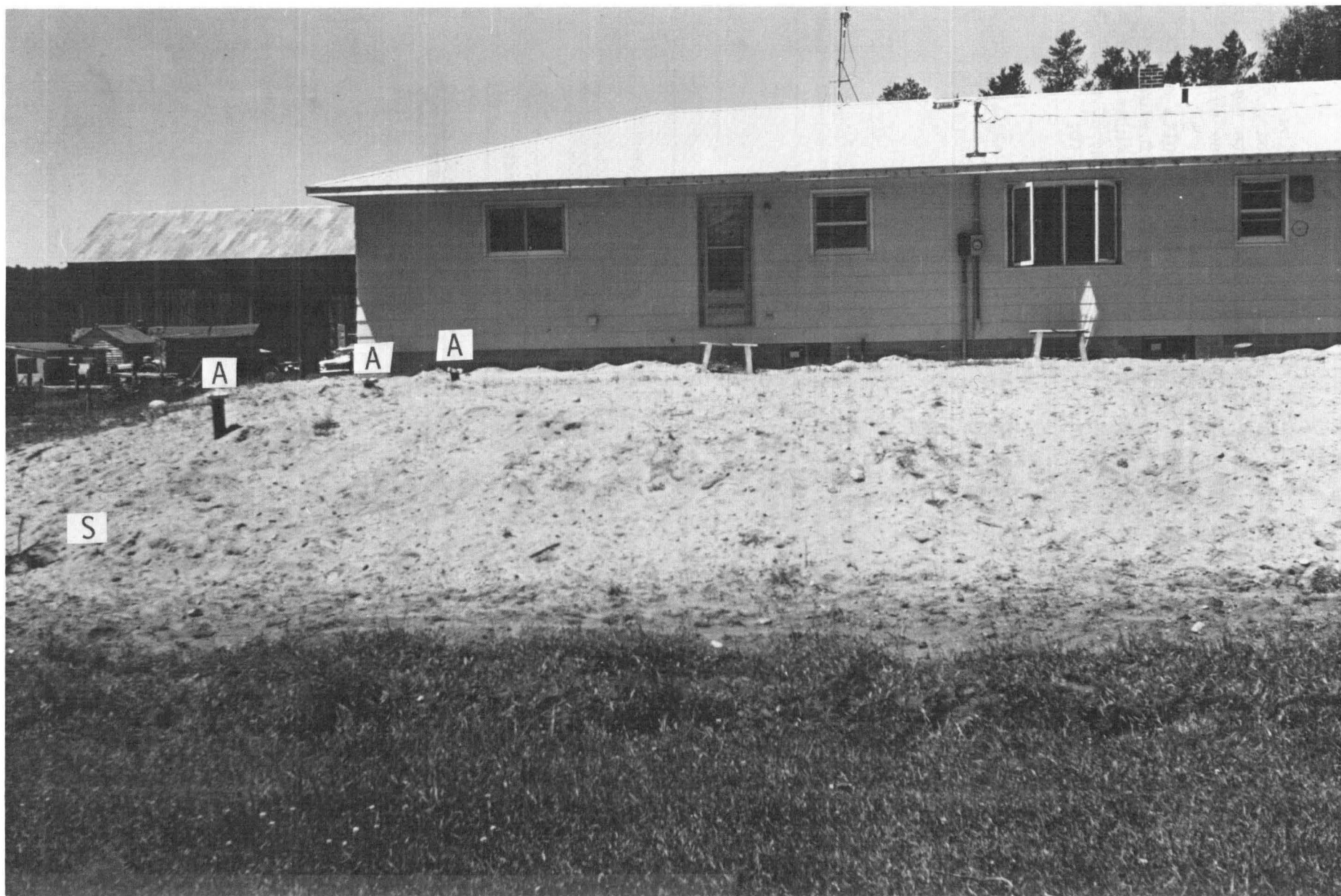
Photo 8.1. Mound System 1 (Clark County) (summer 1970). Effluent seeped through the side of the unfinished mound at point S in early June 1970. Air vents (A) are at the ends of the three tile lines (see diagram of system, Figure 8.3.3).
