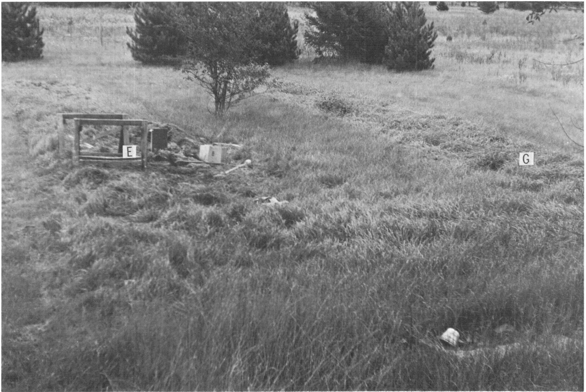
Photo 5.2. Absorption field in Plainfield loamy sand (system 1). The location of the seepage beds, which were partly filled with effluent, is clearly marked by lush growth of grasses (G). An excavation (E) was made next to the middle bed for purposes of sampling and measurement of soil moisture tensions (see diagram, of system, Figure 5.2).
