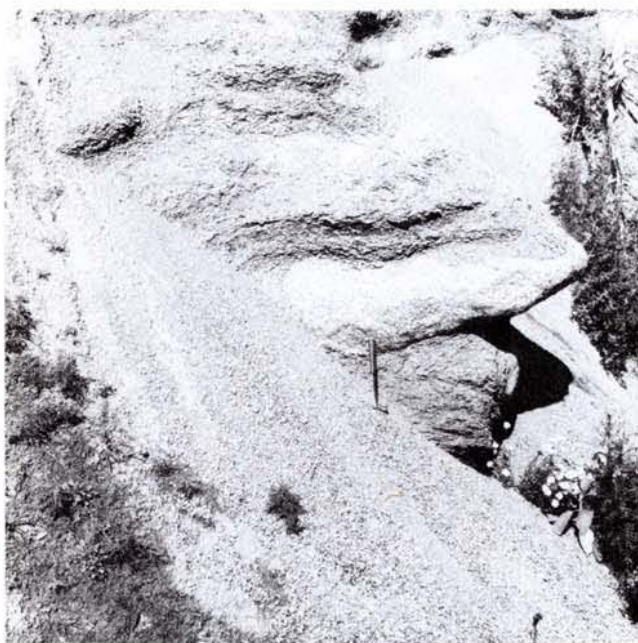
Figure 62.--(A) Grus quarry with near vertical and horizontal joints that control disintegration. (B) Spheroidal boulder in grus pit showing the exfoliation associated with the development of the grus.
