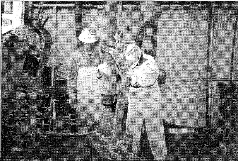
**Figure 3.** March 26, 1992. *Begard Drilling Company of Mt. Pleasant, Michigan, crew adds a joint of 30-ft drill pipe to the drill stem at the 3,900-ft level.*
