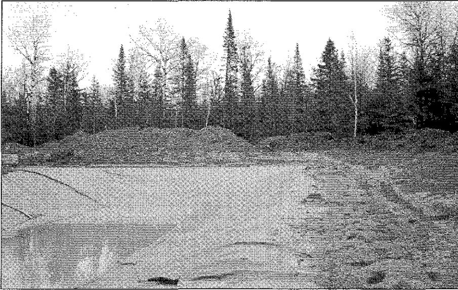
**Figure 2.** March 8, 1992. A part of the drilling site was occupied by this 1,850 cubic yard maximum capacity drilling fluid (mud) pit, composed of 40-mil-thick lining made of PVC resin.
