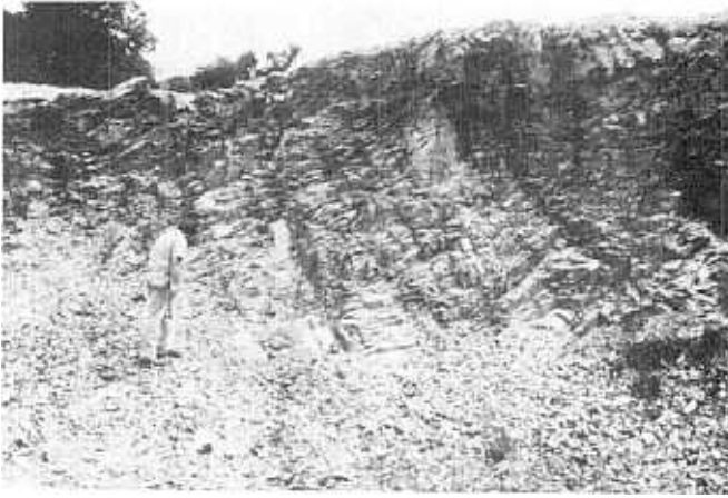
Figure 3. Excavation face at Hamilton Mound quarry showing steeply dipping beds in quartzite cut by nearly horizontal fracture cleavage.
