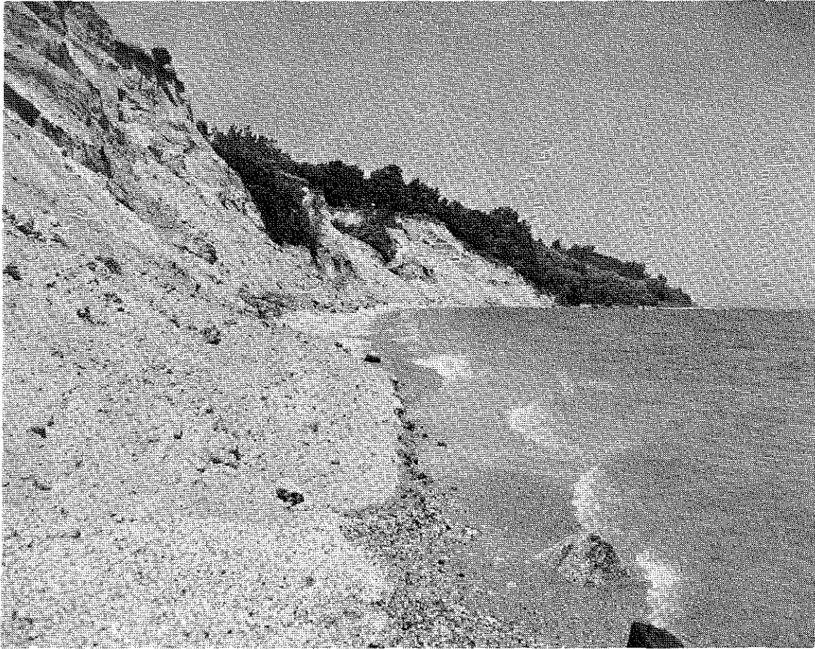
Figure 14. The section of shoreline in the background has been protected by the groins shown in Figure 13. By interrupting the flow of sand along the shore, however, these groins have also contributed to the accelerated erosion of the shoreline shown in the foreground.
