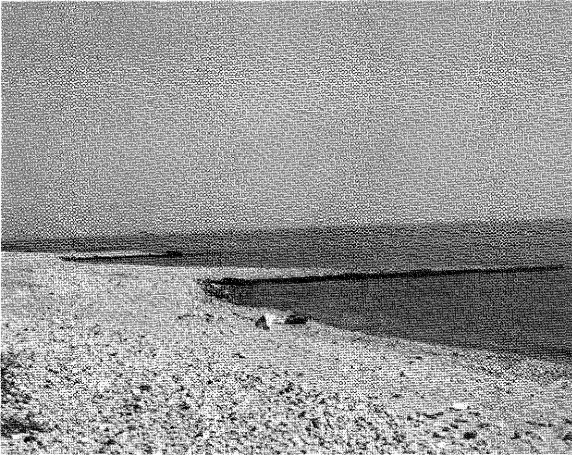
Figure 13. Groins interrupt the flow of sand being carried along the shoreline by the littoral drift. The resulting beach protects the shoreline.
