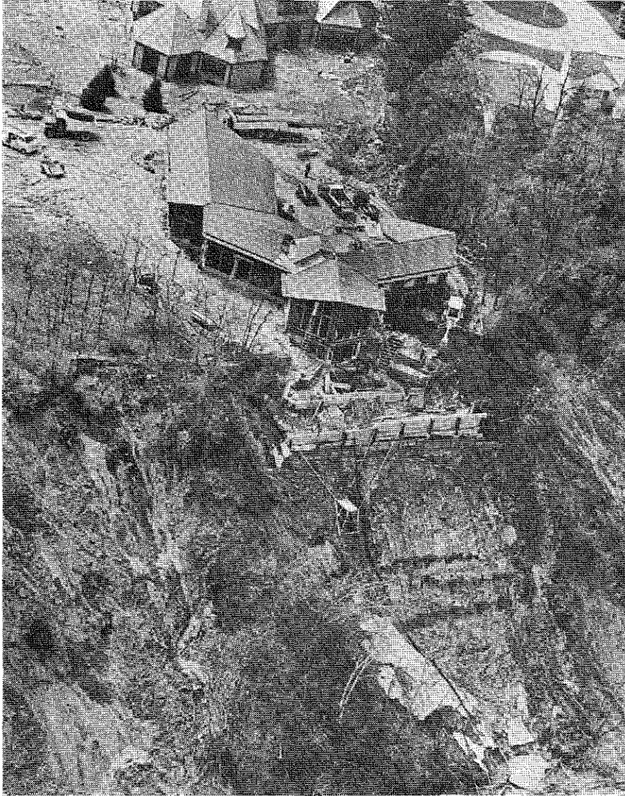
Figure 17. The scars of recent landslides show that this home is being built near the edge of a high, unstable, and actively eroding bluff. Zoning ordinances are needed to protect the unwary citizen. (Milwaukee Journal Photo)
