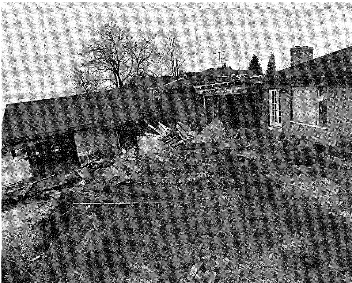
Figure 16. Attempts to protect this residence have obviously been unsuccessful. (Milwaukee Journal Photo)
