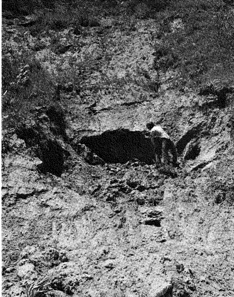
Figure 10. Springs such as this form where the groundwater moving downward through the bluffs encounters a zone of low permeability. Groundwater seepage plays an important role in the retreat of the bluffs along much of the Lake Michigan shoreline in southeastern Wisconsin.
