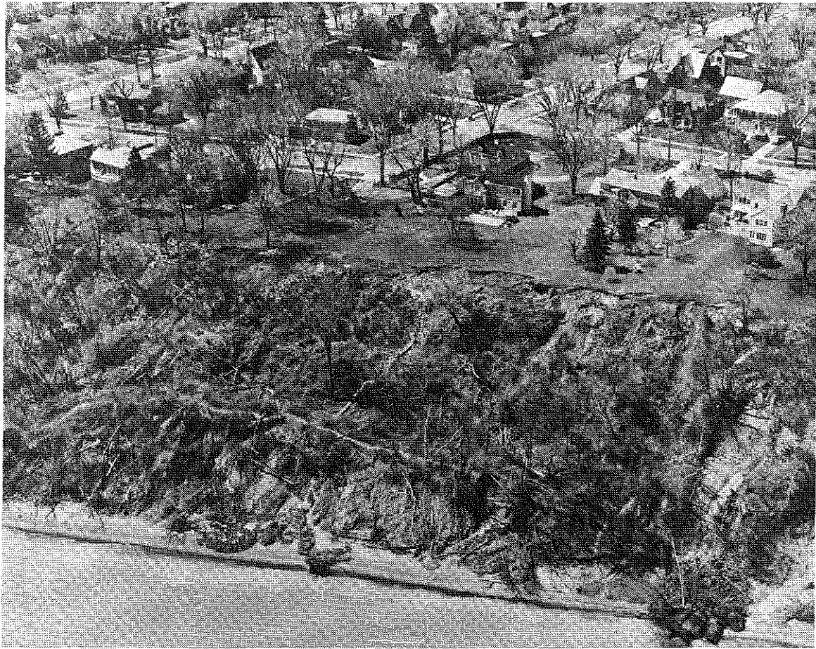
Figure 9. Continuing erosion at the toe of the bluff has caused a series of slumps to occur along this section of the shoreline. (Milwaukee Journal Photo)
