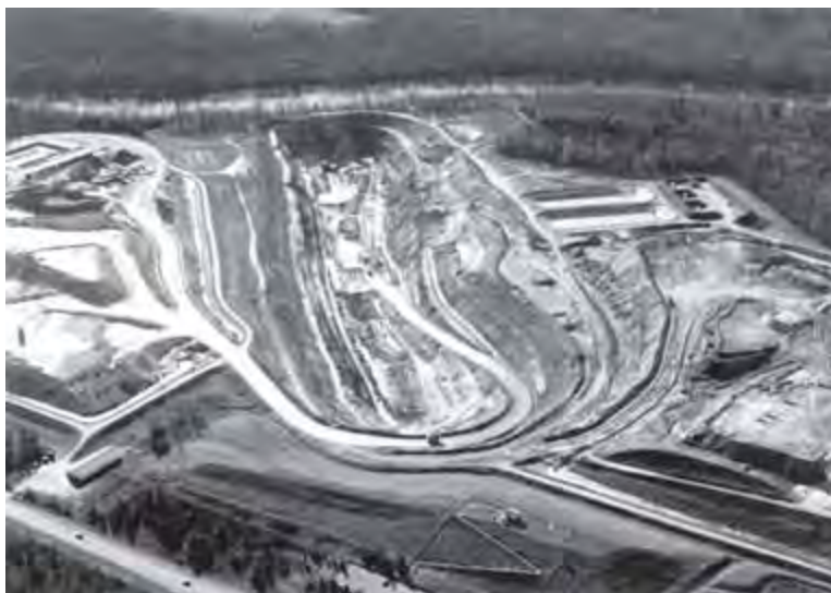
Mining metallic minerals in northern Wisconsin may involve open-pit mines, such as the Flambeau Mine near Ladysmith (photograph circa 1995; site now reclaimed; see p. 19 for a photograph of the reclaimed site) or underground mines, such as the formerly proposed Nicolet Mine in Forest County. Photograph courtesy of Wisconsin Department of Natural Resources.
