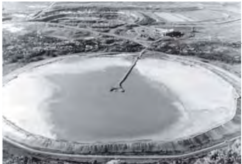
The 320-acre tailings basin at Jackson County Iron Mine was used for the disposal of finely ground rock particles from the mill processing of iron-bearing ore. Mine-waste-disposal facilities regulated under ch. NR 182, Wis. Admin. Code, include those for waste rock, tailings, and all other refuse produced in a mining operation.
