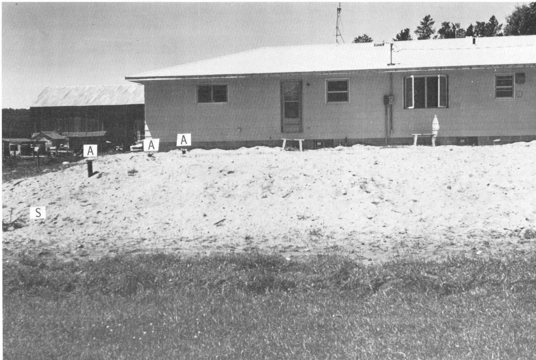
Photo 3.6.3 Mound System II. (unfinished).
