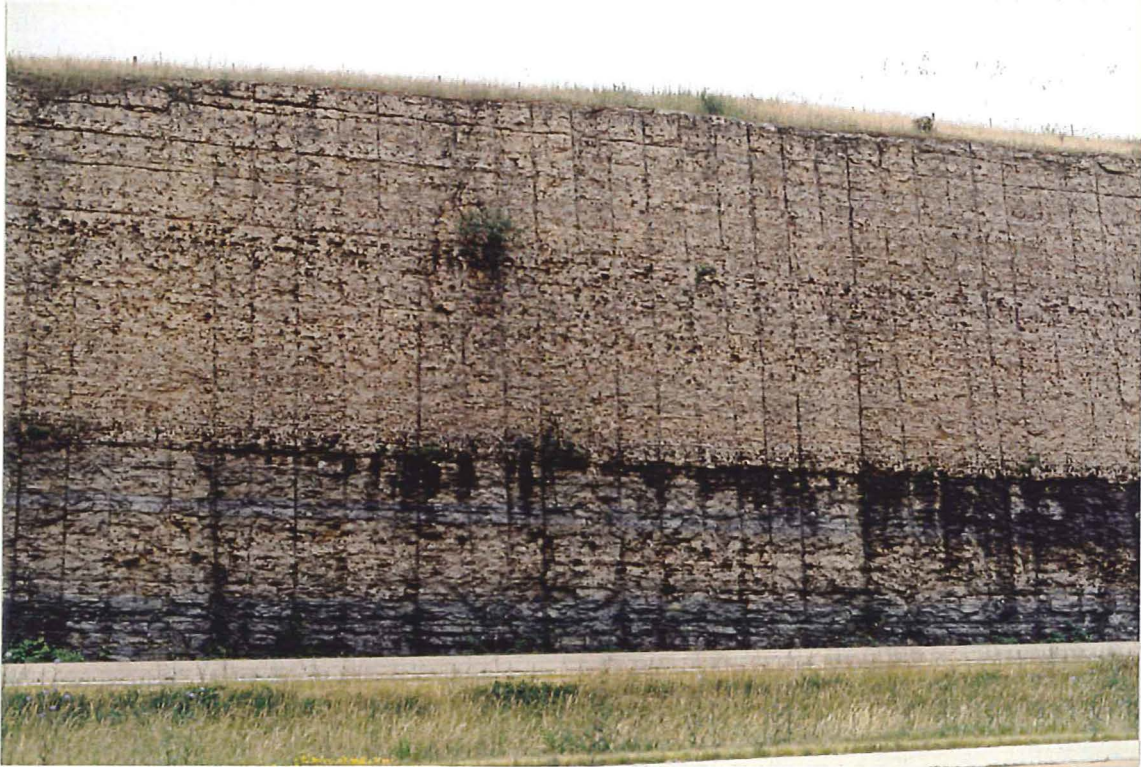
Figure 9. Typical lower Galena of southwestern Wisconsin, exposed in road cut on Hwy 151 east of Barneveld, Iowa County. The lon is the darker interval below the prominent bedding plane marked by water seepage. Dark gray beds at base of cut are shaly dolostone of the Guttenberg Member of the Decorah. Note buff color and pitted weathering typical of overlying Dunleith Member.
