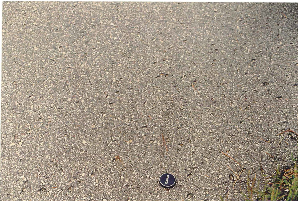
Figure 1 Pitted surface of asphalt pavement on Hwy 18 west of Montfort, Iowa County. Surface pits are caused by deterioration of aggregate particles under exposure to weathering for approximately one year. Lens cap is approximately 2 inches wide.
