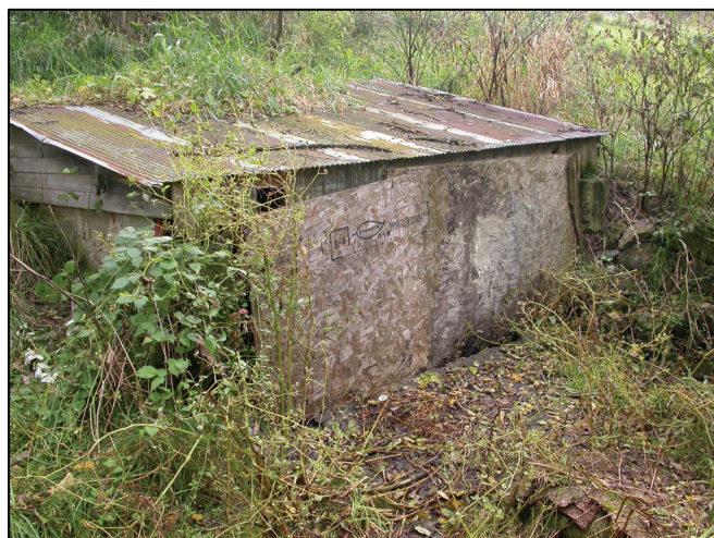
Figure 4. A deteriorated springhouse. The spring beneath this structure, flowing at 120 gallons per minute (0.27 CFS), once supplied water to the inhabitants of a nearby farm.
