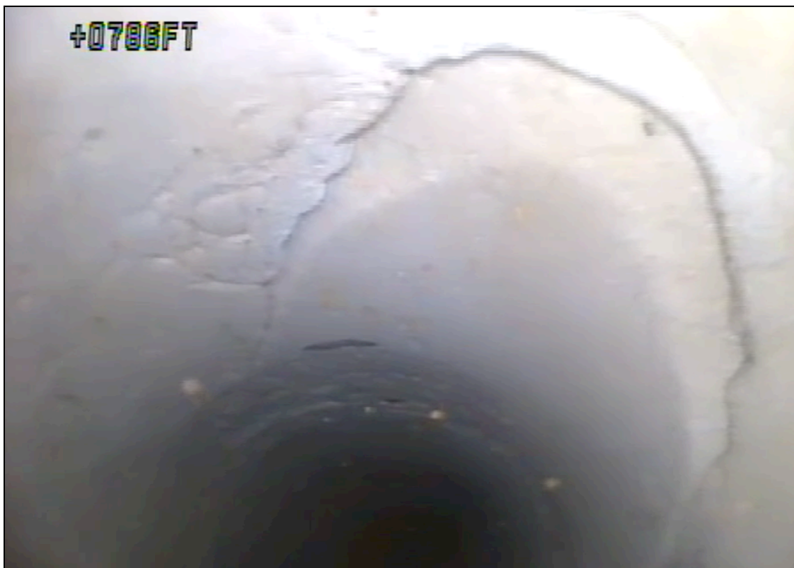
Figure 8. Parabolic fracture at depth of 786 feet in Shorewood Golf Course well (BN-422), Green Bay, Wisconsin.
