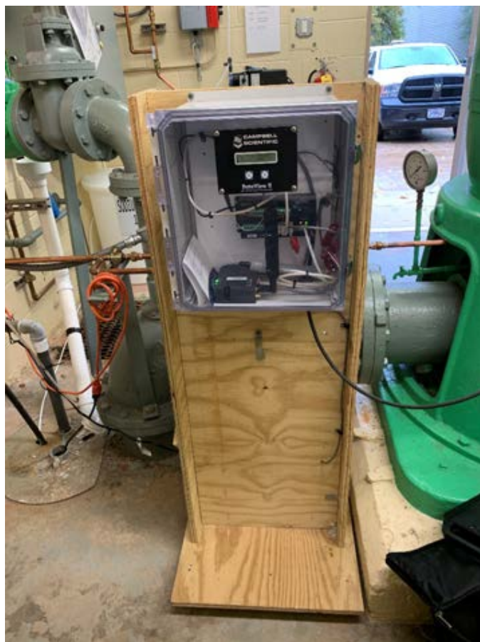
Figure 13. BN-99 retrofitted with a vented submersible pressure transducer with datalogger and digital readout, newly installed on July 14, 2020. The well is test pumped monthly and water-quality samples are collected quarterly in satisfaction of state well codes. Photo courtesy of U.S. Geological Survey.
