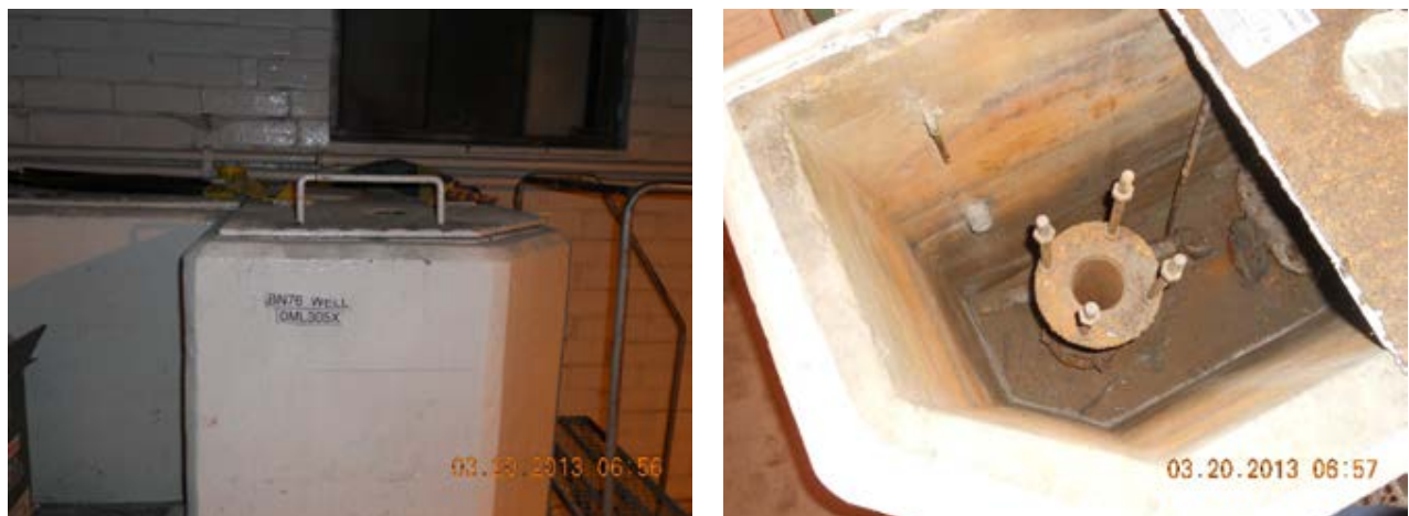
Figure 9. Well BN-76 located in the basement of a privately owned power plant; well shelter (left) and well head (right). Photos courtesy of U.S. Geological Survey.
