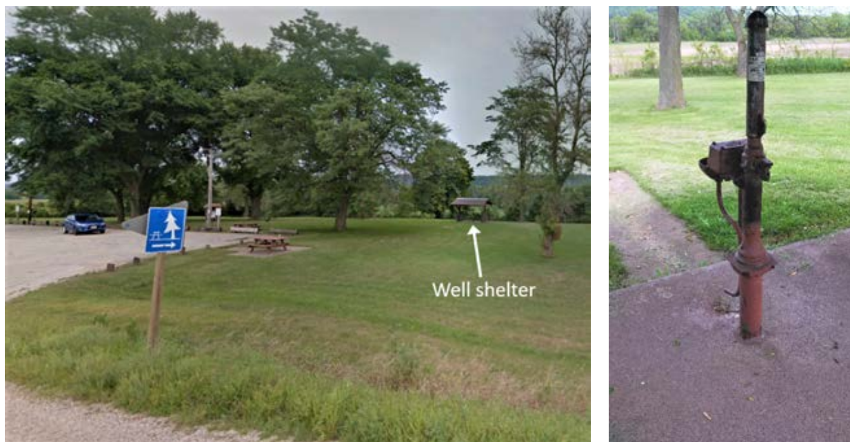
Figure 83. TR-71 located under a shelter at the WisDOT wayside along U.S. Highway 53 (left) and a close-up of the inoperable hand pump prior to removal (right).
