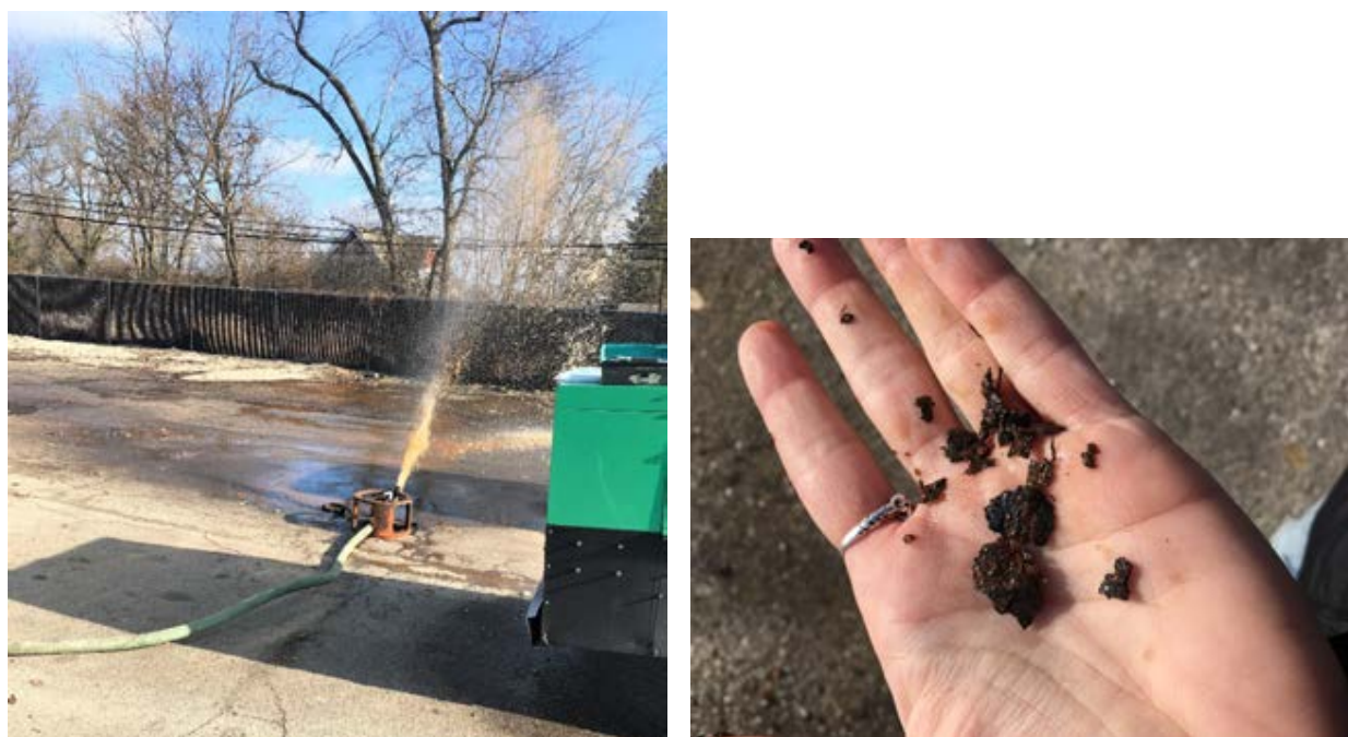
Figure 57. (Left) Debris airlifted from ML-148 on December 3, 2019. Note the discoloration of the water due to the removal of biofoul build-up along the borehole wall. (Right) Pieces of disintegrated and rusted metal casing that were air lifted from well during development.
