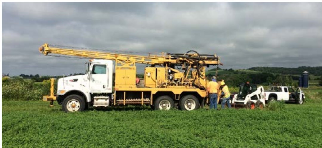
Figure 37. Drill rig on site preparing to drill IW-3623, the replacement for IW-32. Well drilling was completed August 14-16, 2019.
