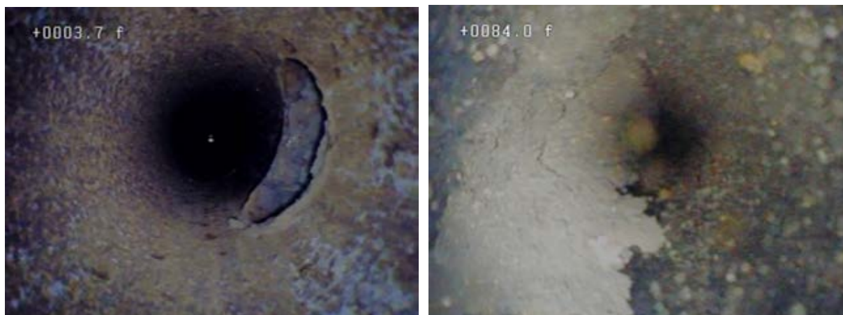
Figure 48. Still shots from borehole video log of ML-118, collected on November 7, 2018, showing a hole in the casing wall (left) and a large amount of biofilm and debris in the well (right). The camera stopped at a blockage around 104 ft bls (as measured by video cable).
