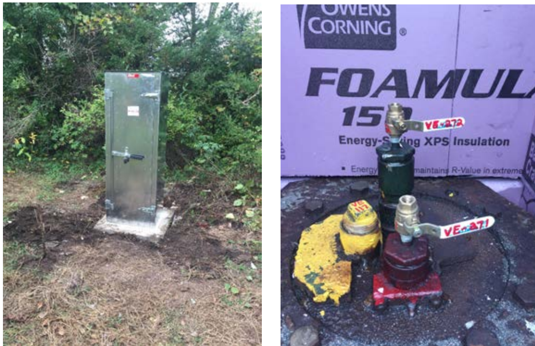
Figure 89. New insulated and heated monitoring shelter (left) and new piezometer heads for VE-117, VE-271, and VE-272 in the shelter (right). Work was completed in November of 2019. Photos courtesy of U.S. Geological Survey.
