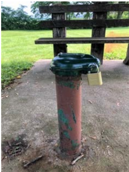
Figure 85. Newly installed wellhead with cover and lock for well TR-71.
