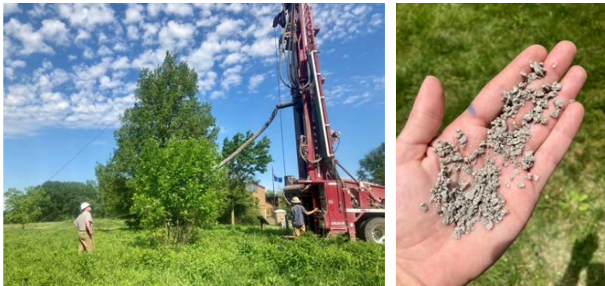
Figure 50. Drilling ML-8035 (left) and carbonate bedrock cuttings (right).
