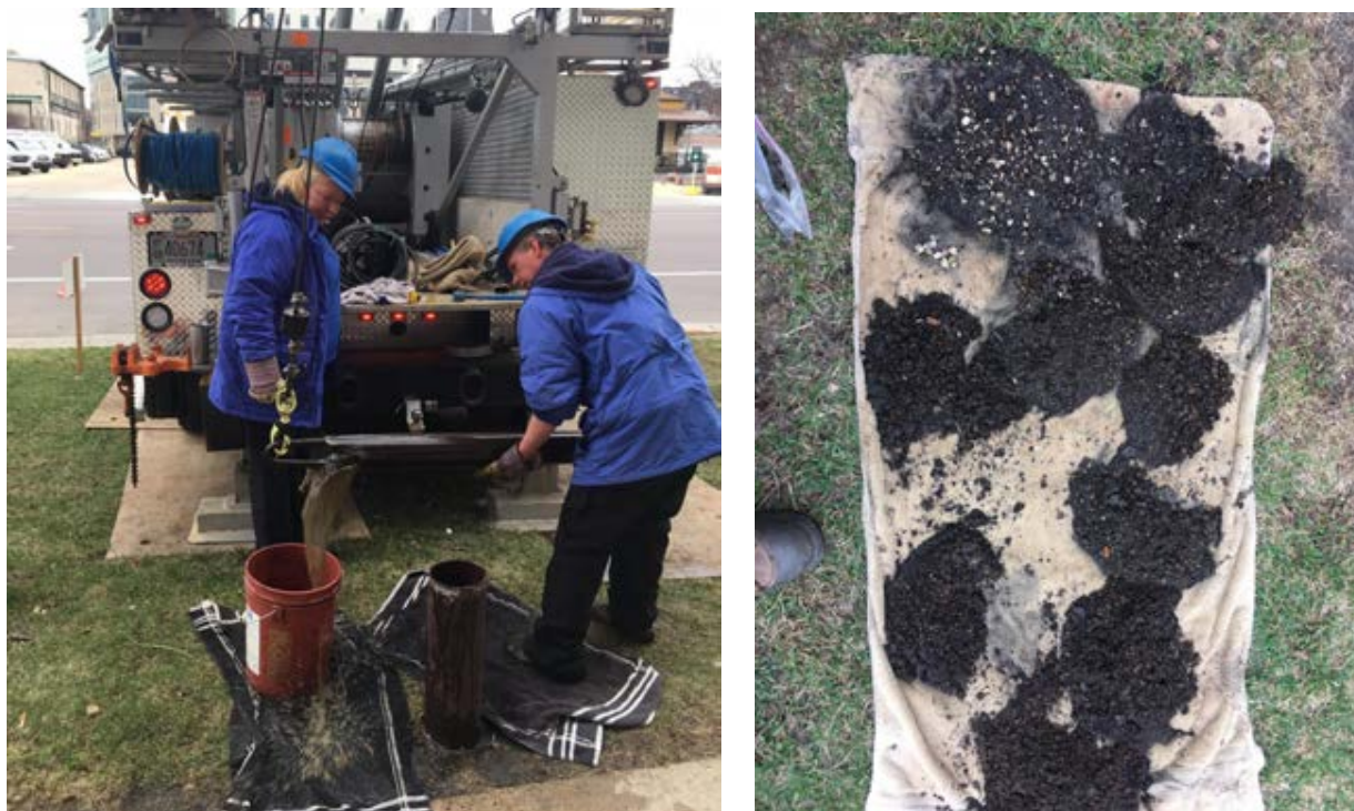
Figure 27. Using a bailer to remove debris and redevelop DN-1297 (left) in the spring of 2019. Cement and other material removed from the bottom of the well (right).
