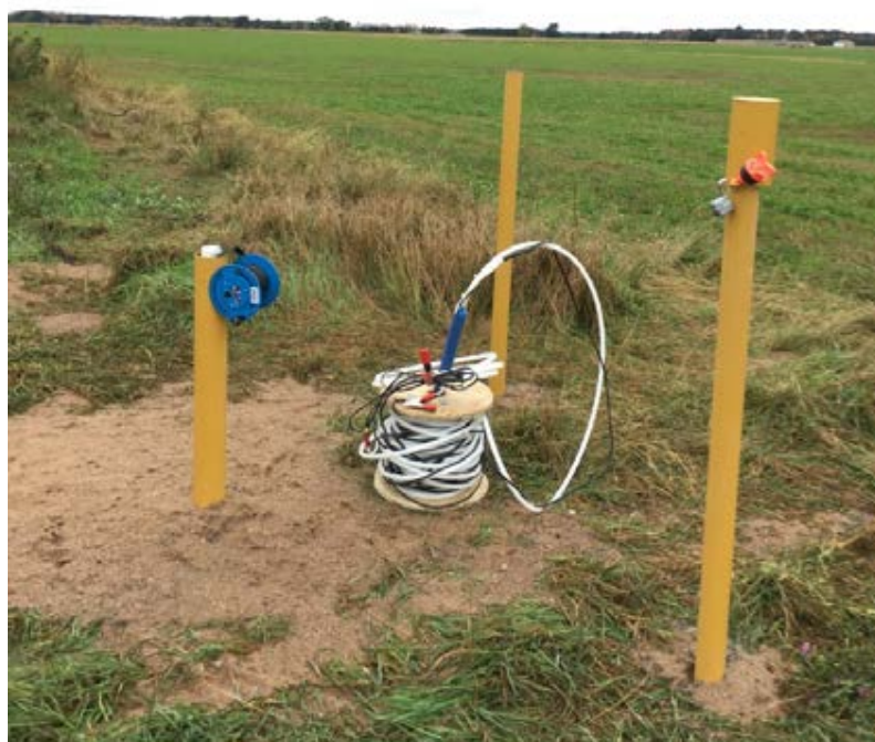
Figure 43. Newly completed well LA-1493 with white 2-in.-diameter PVC well casing visible above the 4-in.-diameter protective cover pipe (left-most yellow post). Two high-visibility protective bollards are located to the right of the well. A submersible pump, equipped with tubing for developing the well, is visible on the ground and an electronic tape for taking discrete tape-down measurements is hanging from the well head.
