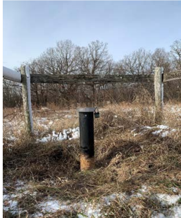
Figure 92. New locking wellhead (left) after old equipment was removed and well WK-31 after old shelter was removed. All work was completed by December 2020. Photos courtesy of U.S. Geological Survey.
