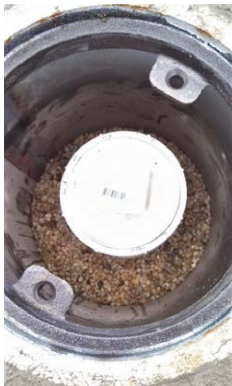
Figures 56. ML-148 flush-mounted protective well cap (left) and PVC well head located below ground surface within a steel protective cover flush-mounted with the parking lot (right). Photos courtesy of U.S. Geological Survey.
