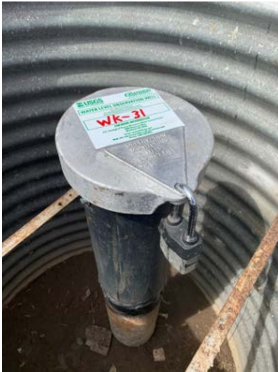
Figure 92. New locking wellhead (left) after old equipment was removed and well WK-31 after old shelter was removed. All work was completed by December 2020. Photos courtesy of U.S. Geological Survey.
