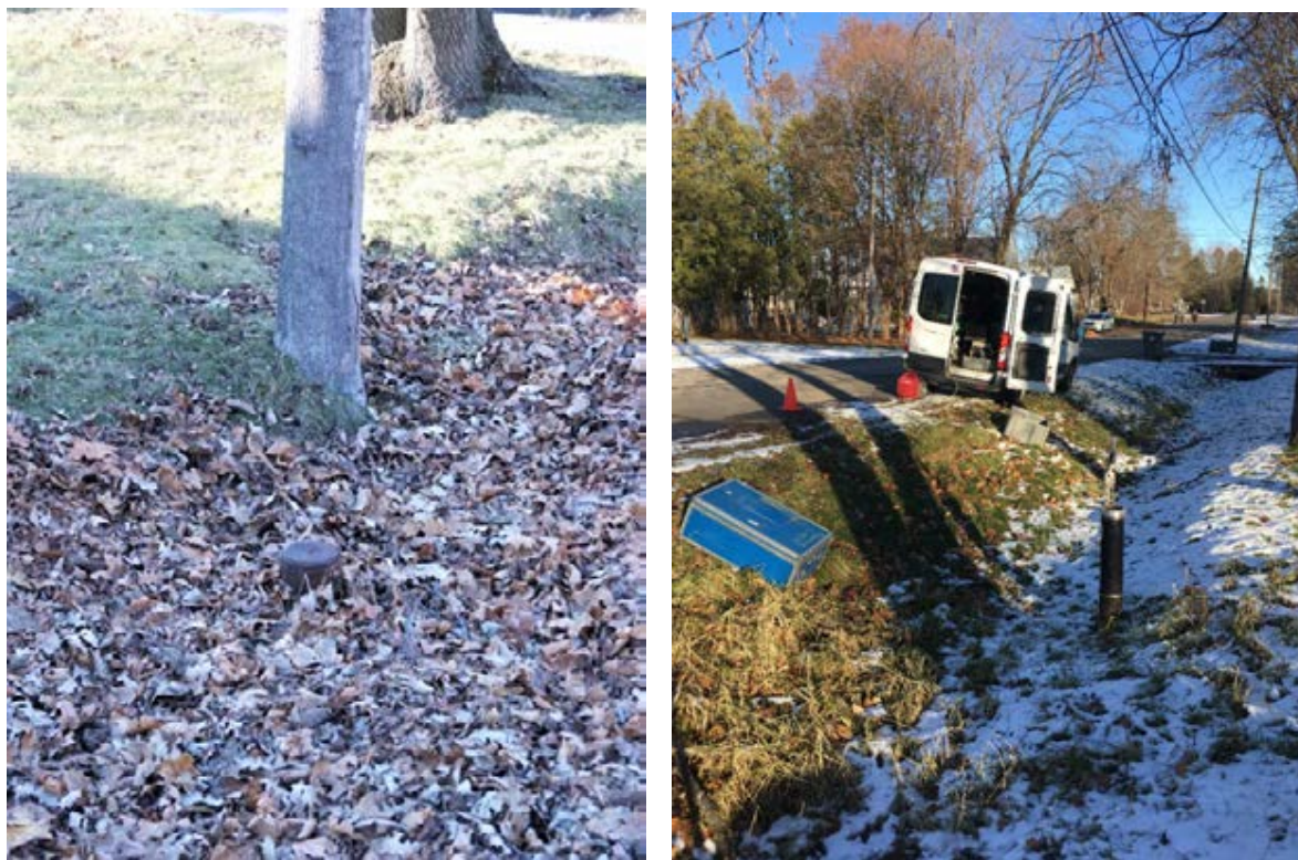
Figure 73. The MQ-09 well head, located just inches above grade, in a drainage ditch (left) and after an extension pipe was welded on (right). The WGNHS geophysical logging van is present in the background (right). Photo on left courtesy of U.S. Geological Survey.
